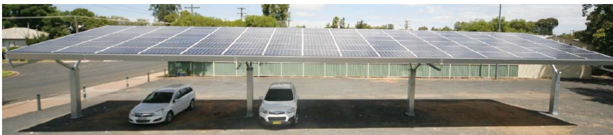
Figure 5.10 PowerPark shade structures to provide car parking cover and solar power
